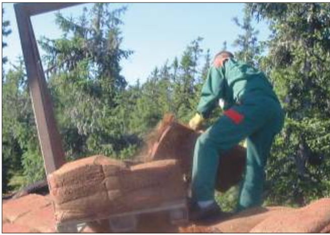
Easy to lift up on the roof: Each bag is approximately 17 kg pr. mesh bag or approximately 400 kg pr. pallet.
