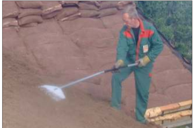
At the end the roof is evened with peat before watering.
