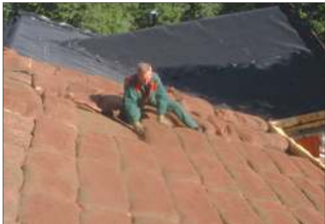
Lay the mesh bags close together.
