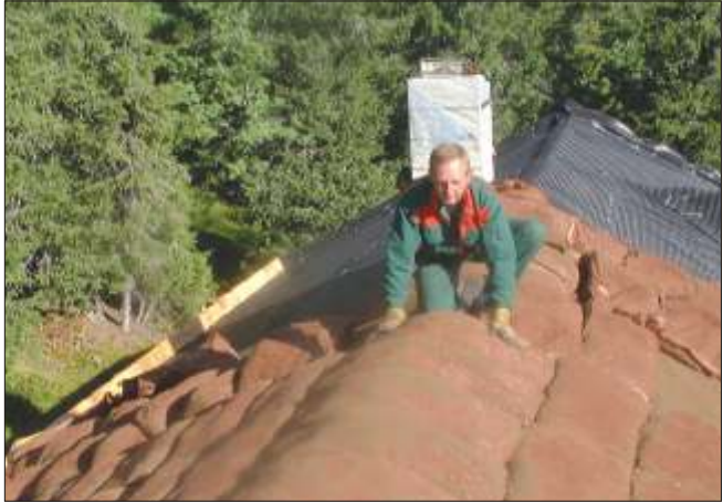
The mesh bags should be laid across the roof top.
