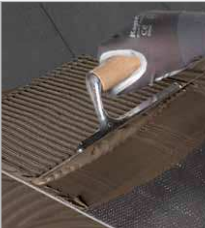
Fig. 7.2 - laying on floors: spreading the adhesive on the back of the tile
