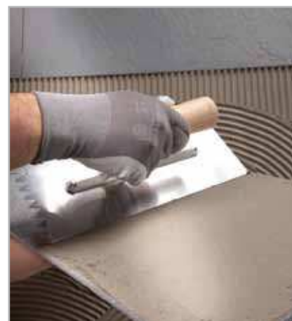
Fig. 7.5 - Fixing to walls: applying the adhesive on the back of a tile Note. Image does not match text
