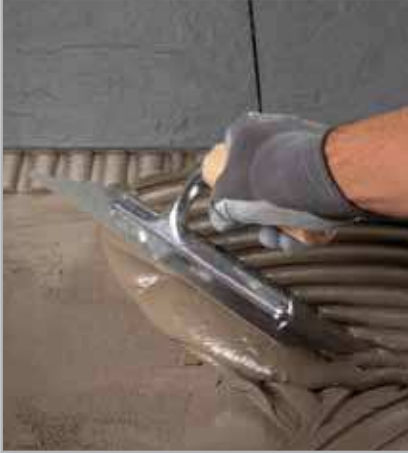
Fig. 7.1 - Laying on floors: spreading the adhesive with a round-toothed 9 mm radius notched trowel
