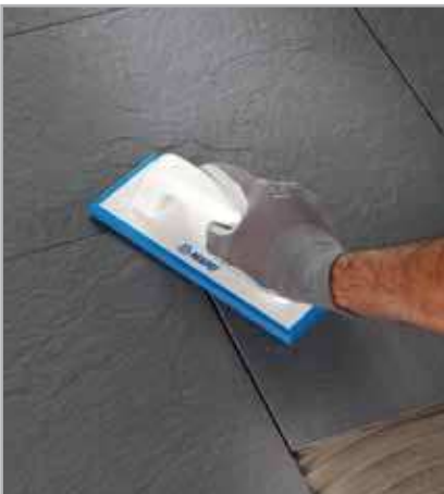
Fig. 7.3 - Laying on floors: laying and tapping the tiles in place
