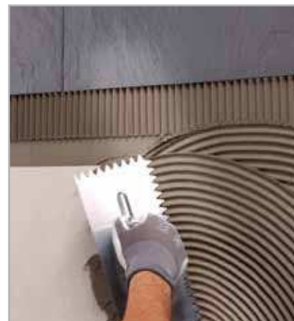
Fig. 7.4 - Fixing to walls: spreading the adhesive with a N° 6 notched trowel Note. Image does not match text
