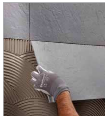
Fig. 7.6 - Fixing to walls: positioning a tile Note. Image does not match text
